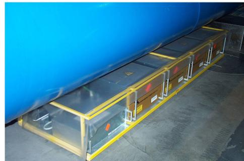
Figure 3: Protection rack type DYPB installed underneath the main dipoles.
